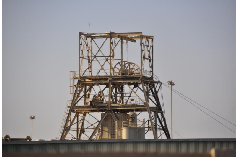
Above-ground Constructions at Ezulwini's Underground Mine
