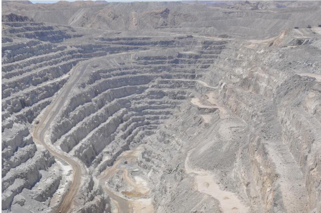
The Open Pit of Rössing Uranium Mine, Namibia. (Size: 3000 m x 1000 m x 400 m, l x w x d) Picture taken by D.H. Trampé, 2010. Picture used with kind permission of the photographer.
