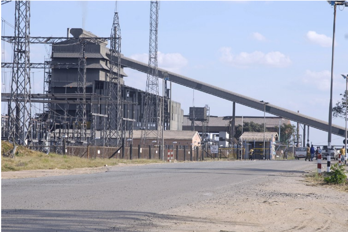
Chambishi Metals' COSAC plant. The company used to enjoy a good standing among Zambians, but several accidents have occurred during 2007, seriously wounding workers. Photo: Petter Bolme, Global Reporting.
